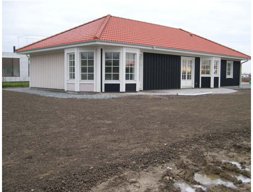
Facade mod have.
